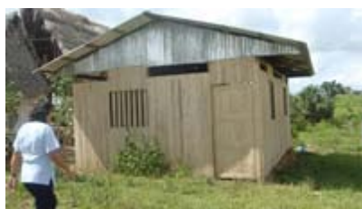
First Casa de Espera awaiting interior finishing
